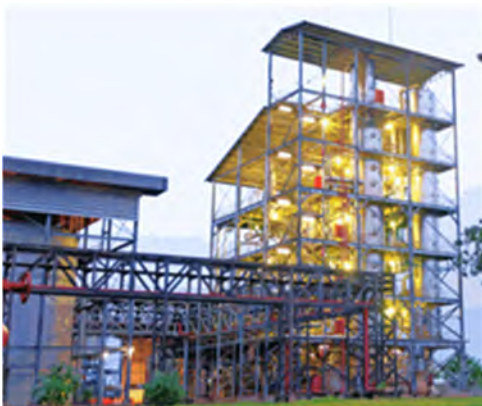
Exhibit 78: BBE ethanol plant
